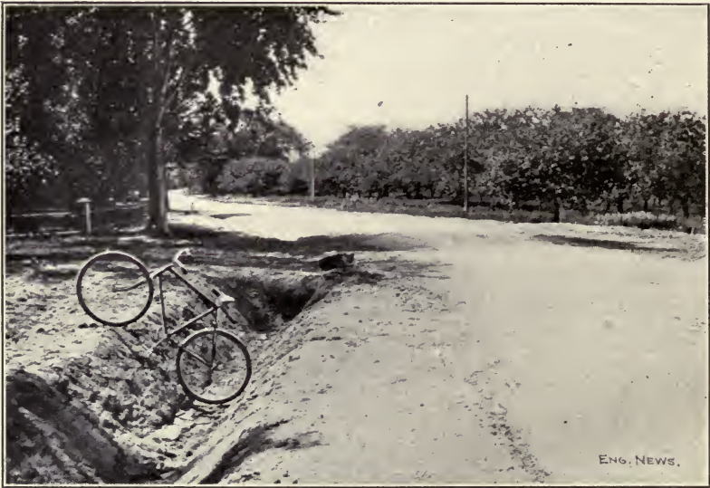
FIG. 3.—MACADAM ROAD WITH DEEP DITCHES
